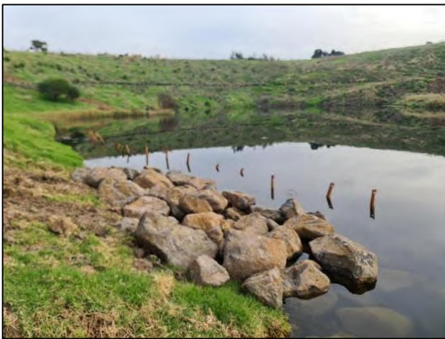
Plate 15. Rock beaching within the offset area (Ecology and Heritage Partners Pty Ltd 15/06/2022).
