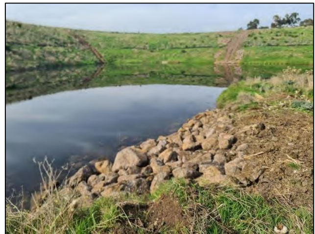
Plate 16. Rock beaching within the offset area (Ecology and Heritage Partners Pty Ltd 15/06/2022).
