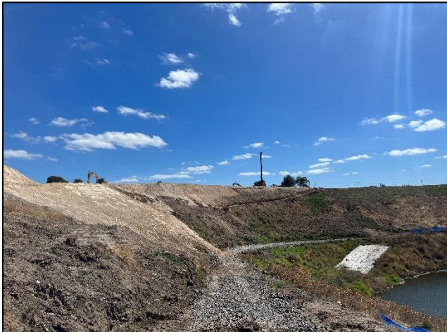
Plate 1. Access track to offset area with backfilling and piling being undertaken, and jute matting laid (Ecology and Heritage Partners Pty Ltd 14/02/2023).
