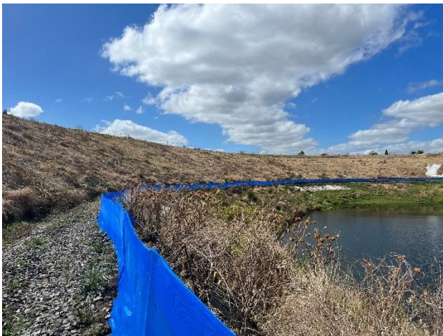
Plate 12. Frog exclusion fencing installed around offset area 1 (Ecology and Heritage Partners Pty Ltd 27/04/2022).
