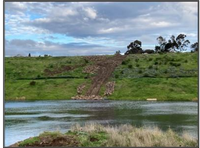
Plate 9. Rock beaching and habitat improvement works underway in offset area 1 (site 1) (Ecology and Heritage Partners Pty Ltd 26/04/2022).
