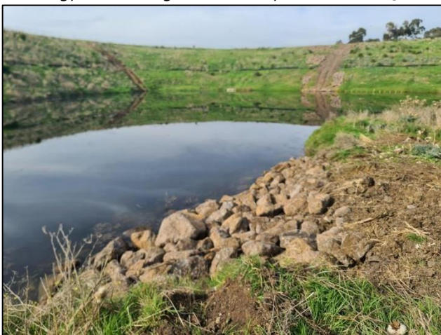
Plate 5. Rock beaching within the offset area (Ecology and Heritage Partners Pty Ltd 15/06/2022).
