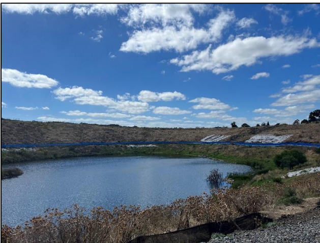
Plate 3. The north-west area of offset area where backfilling and piling undertaken, and jute matting laid (Ecology and Heritage Partners Pty Ltd 14/02/2023).
