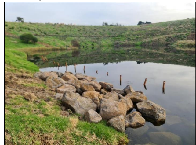
Plate 4. Rock beaching within the offset area (Ecology and Heritage Partners Pty Ltd 15/06/2022).
